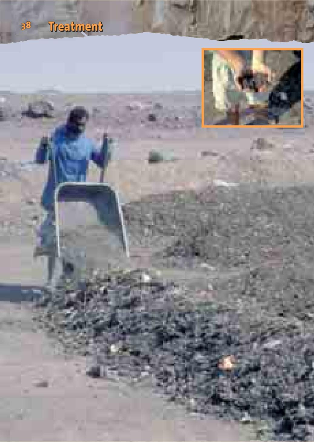
Composting is an aerobic process in which bacteria and other organisms feed on organic material and decompose it. Composting (one material) and co-composting (two or more materials) represent generally accepted procedures to treat excreta.
