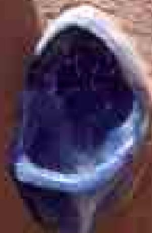
Waterless urinals, slab or wall-mounted, collect undiluted urine, and so generate relatively low volumes. Traditionally urinals are provided adjacent to a toilet. Urinals can prevent fouling of toilets, especially in schools.
