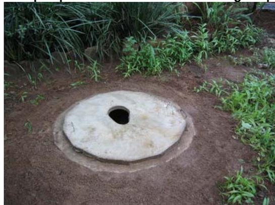
The slab is then brought close by. A layer of clay, cement or termite mortar is then laid on the ring beam, The slab laid centrally on the ring beam. Now the superstructure must be built around the slab.
