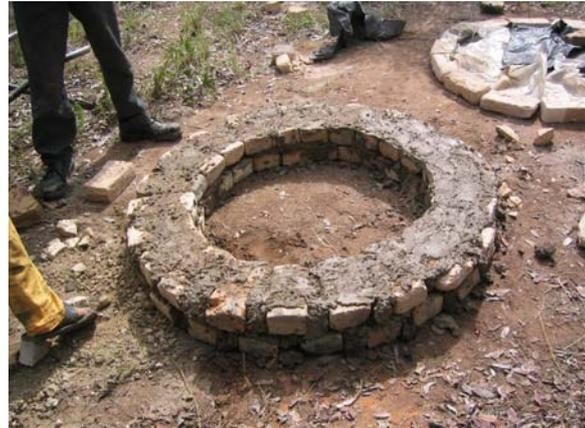
The brick ring beam is bonded together with anthill mortar, in between and above the bricks. Two courses of bricks are laid, one above the other and placed so that the upper bricks lay over the joint between the lower bricks. (note - if bricks are not available a concrete ring beam can be made instead).
