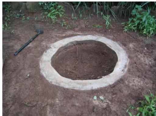
The site of the toilet is first levelled off with a hoe and the rim beam placed firmly on the ground. The hole is then dug inside the ring beam down to a depth of 1 to 1.5 metres. Some of the excavated soil is placed around the ring beam and rammed in place. This will help to prevent rain water undermining the pit.
