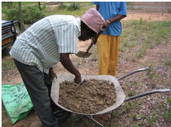
A suitable site for the toilet is located, preferably on slightly raised ground. A circle is marked on the ground 80cm in diameter. A ring of fired bricks is laid on the chosen site around the mark to start making the ring beam. Anthill mortar is gathered, broken up and mixed with water to make a stiff mortar.
