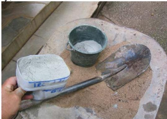
A measuring device can be made with a 2 litre plastic milk bottle cut in half. Measured amounts of water are added and marks made on the bottle. When full the measuring device holds one litre of material. A mark showing half a litre is also shown. For this slab 5 litres of cement is mixed with 30 litres sand (6:1).
