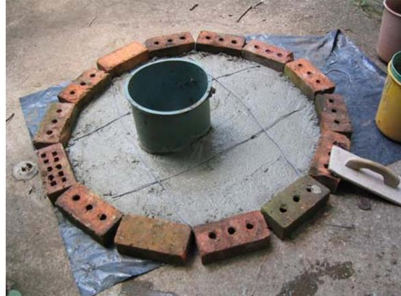
Half the mix is made first with 5 litres cement and 15 litre river sand in a wheelbarrow. The concrete slurry is added to the base of the mould and distributed evenly over the whole surface. The four wires are then added as shown at right angles to each other.
