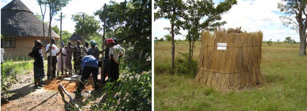
*This house structure is used to make the place private. There are many ways of making the house structure. It is best to make a roof to fit over the structure for shade and to keep the rain out.*
