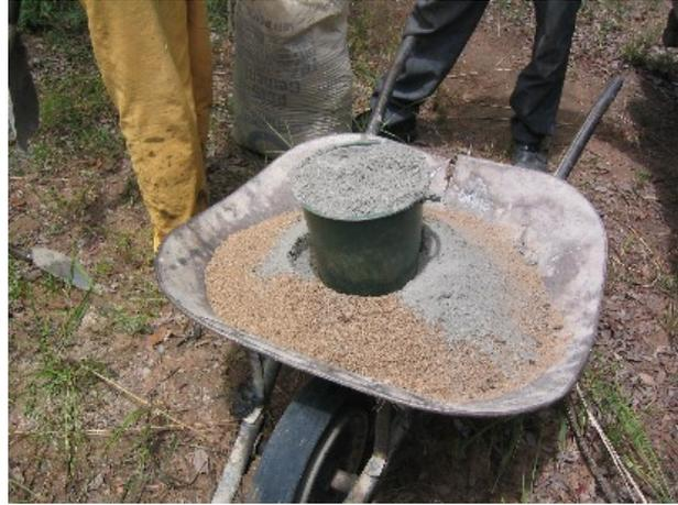
*The sand and cement must be very well mixed. After mixing the dry sand and cement add water (about 2 - 3 litres) to make a stiff mix. Mix thoroughly again. Add half the mix to the slab mould and spread out evenly*
