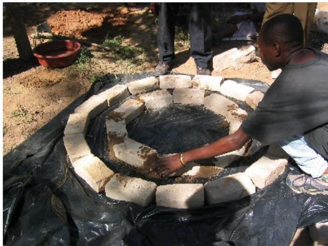
*Once the brick mould has been made, make up the concrete mixture of 5 litres fresh cement with 30 litres good river sand. Mix the dry parts thoroughly first then mix with about 3 litres fresh water. Mix thoroughly again. Add half of this mixture to the mould. Then take a length of 3 – 4mm wire and place above the concrete mix about half way between the inner and outer bricks. Then add the remainder of the concrete mix to the mould and level off with a wooden float.*
