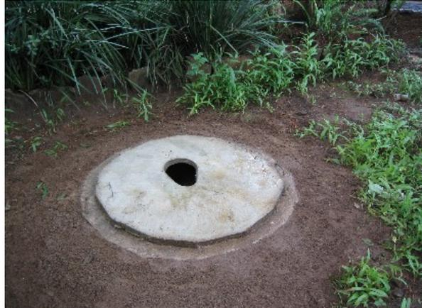
*Dig down hole within the ring beam to at least 1 metre below surface. Place soil around ring beam and ram in place hard. Add leaves to pit base. Lay anthill mortar or weak cement on ring beam and place slab on top. Bed in and level the slab. The structure can now be built around the slab.*
