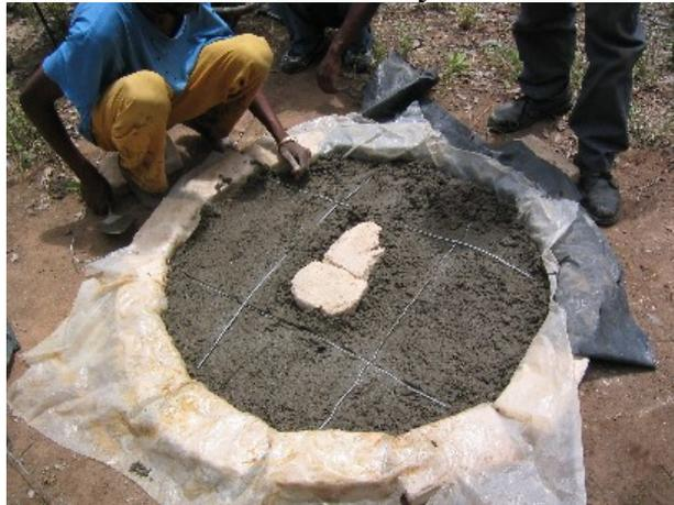
*Add 4 reinforcing wires each 3 to 4mm in diameter and 90cm long in a square shape around the squat hole. Then add the rest of the concrete mixture. Spread out evenly. Also ram down hard with a wooden float. Smooth off with a steel trowel. Add two thick wire handles on either side for lifting.*
