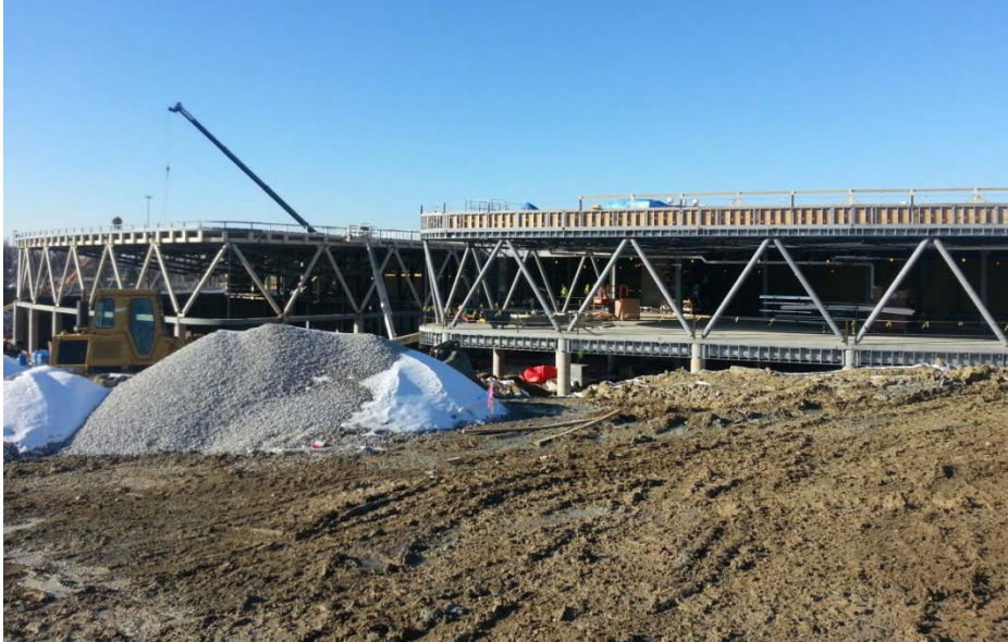
Progress Construction Photo from November 2014
