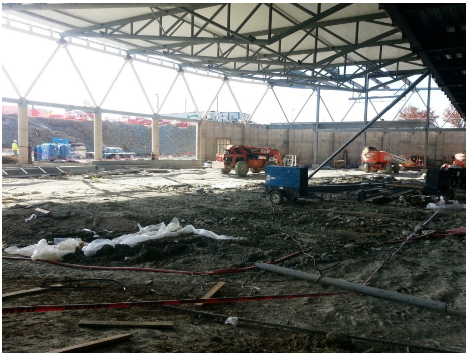
Progress Construction Photo from November 2014
