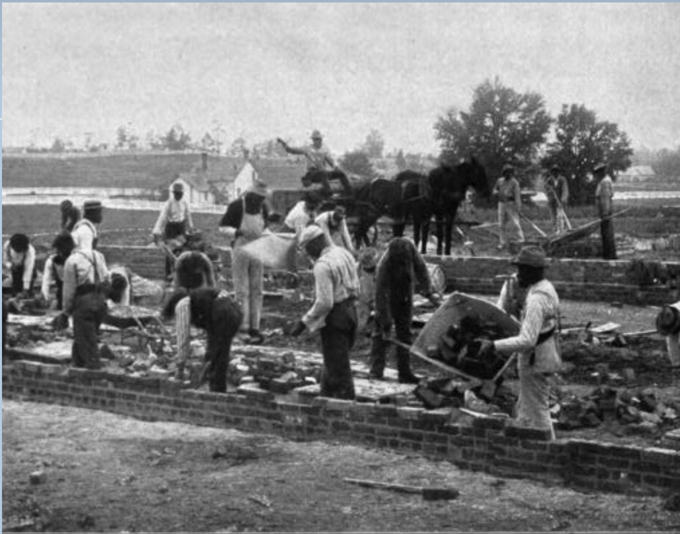
STARTING A NEW BUILDING. Student masons laying the foundation in brick.
