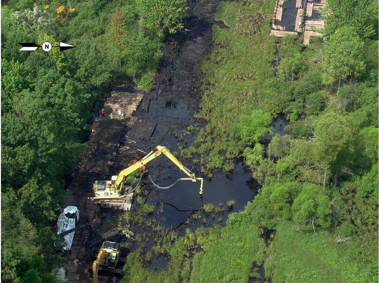
Figure 4. Cleanup efforts in an oil-soaked wetland near the rupture site. Saturated soil complicated the cleanup and excavation efforts. An excavator with a vacuum attachment is shown situated on wooden matting near the rupture site.
